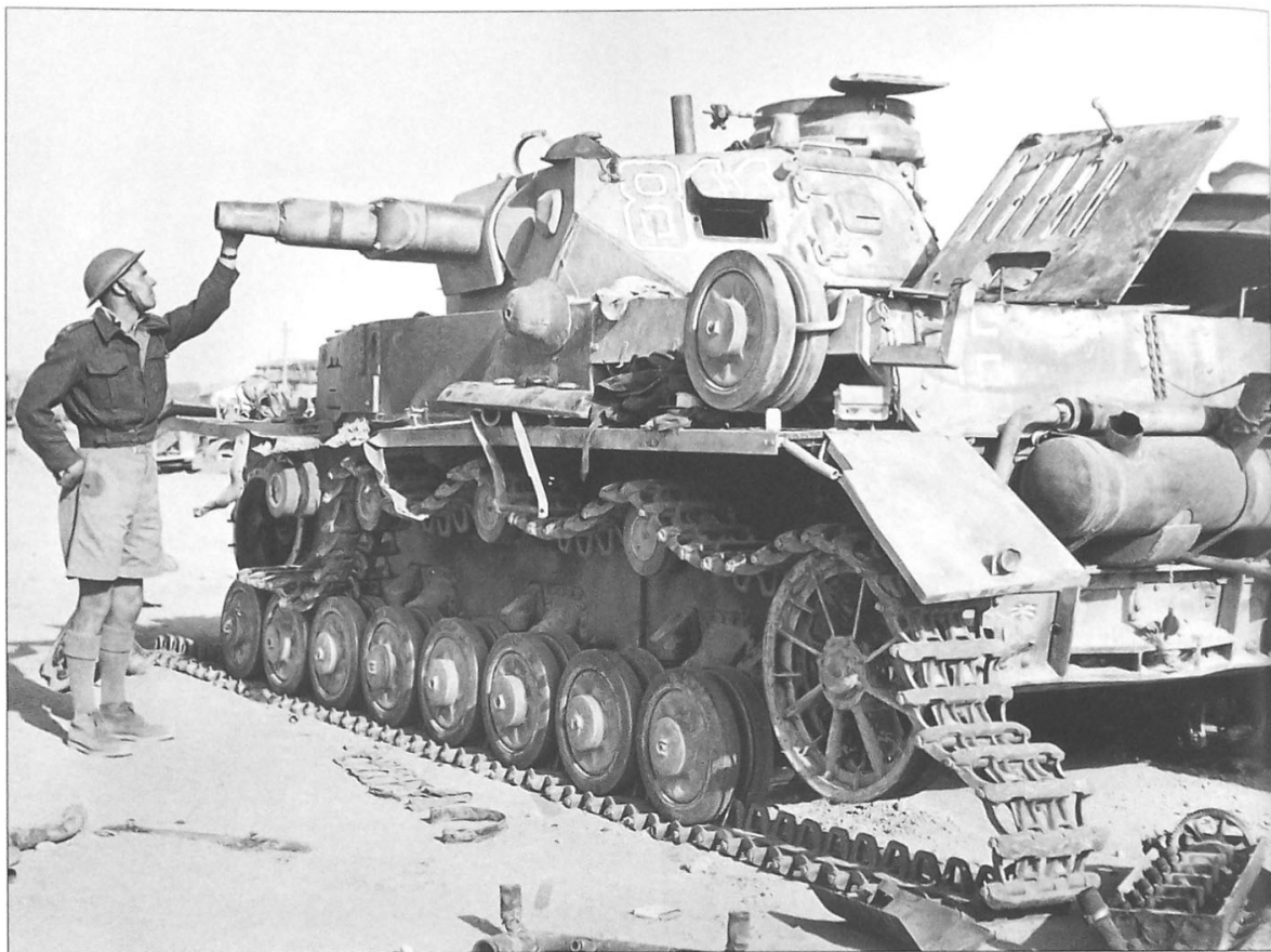
A British soldier examines the 7.5cm KwK L/24 gun barrel of a disabled Pz.Kpfw.IV Ausf.D from Pz.Rgt.5. The vehicle has evidently lost on its tracks, more than likely after receiving an enemy round to its side. Note the engine deck compartment hatch in the open position. A spare road wheel can also be seen attached to the rear engine deck.
