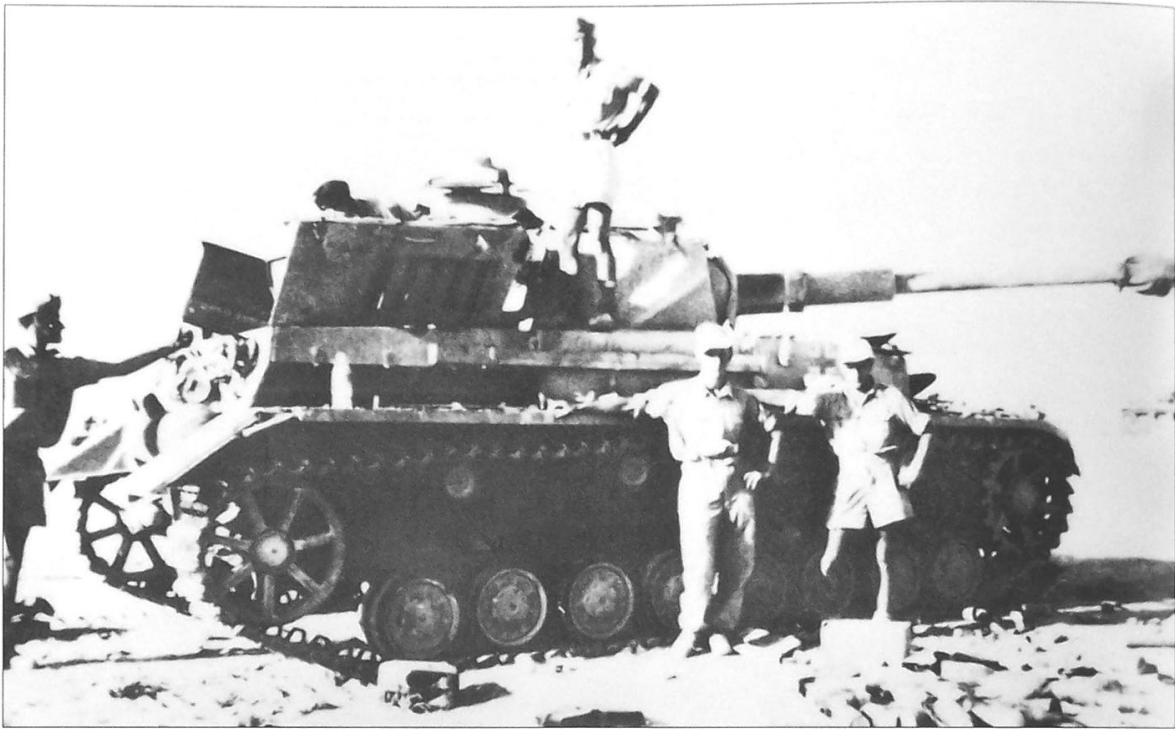
The crew of a Pz.Kpfw.IV Ausf.F2 have halted in the desert following a mechanical fault. The engine compartment doors on the rear deck can be seen fully opened. This tank is armed with the long barrellled L/43 7.5cm gun. Note the protective cover over the muzzle brake of this tank. This was used primarily to avoid any unwanted sand particles entering the barrel when the gun was not in any immediate action. The Pz.Kpfw.IV was probably the most effective and deadliest tank used in the DAK arsenal.
