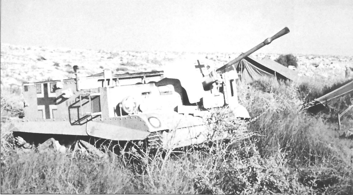
A rare photograph showing a captured Bren Gun Carrier that was modified by the British to mount a 25mm Hotchkiss anti-tank gun. This vehicle is being used by an unidentified DAK armored unit. The Bren Gun Carrier still retains its original dark yellow paint, but the new owners have painted prominent national crosses, which have been applied to the side of the hull and to the front of the gun shield.
