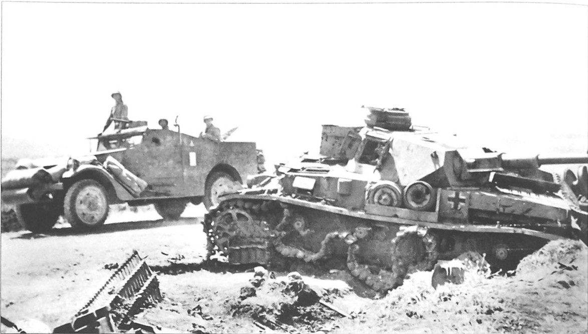
An American White armored scout car passes a destroyed Pz Kpfw IV Ausf. G. The vehicle is armed with a 7.5cm KwK 40 L/48 gun. The tank has obviously received a hit from an anti-tank round, which has consequently led to it losing its track and becoming disabled. The vehicle is painted in overall dark yellow. No other distinguishable markings can be seen except for the small national cross painted on the side of the hull.
