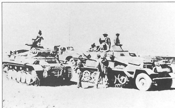
Here a Pz.Kpfw.II Ausf.A-C halts alongside an Sd.Kfz.251 Ausf.B halftrack during operations in the second half of 1941. Both vehicles are more than likely been painted in overall dark yellow to help conceal them from Allied fighters or well concealed anti-tank gunners. The Pz.Kpfw.II is carrying various provisions, and track links have been attached to the front of the hull to help protect its thin armor.
