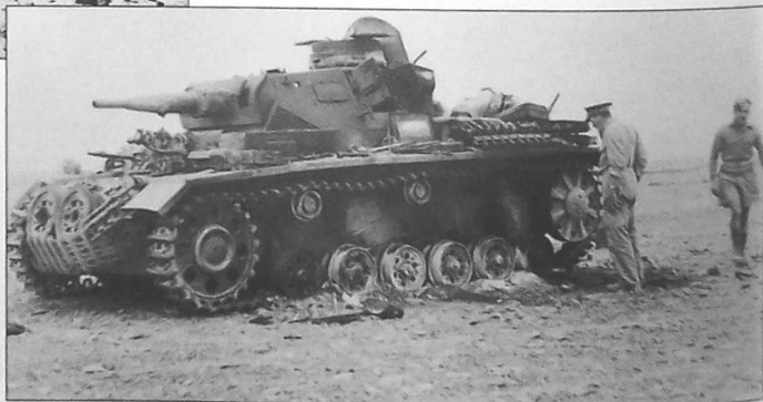
A destroyed Pz.Kpfw.III Ausf.J, which was knocked out of action during the summer of 1942. The tank carries a stowage box on the turret rear, obviously fabricated by the unit's workshops. No markings can be seen on the vehicle.
